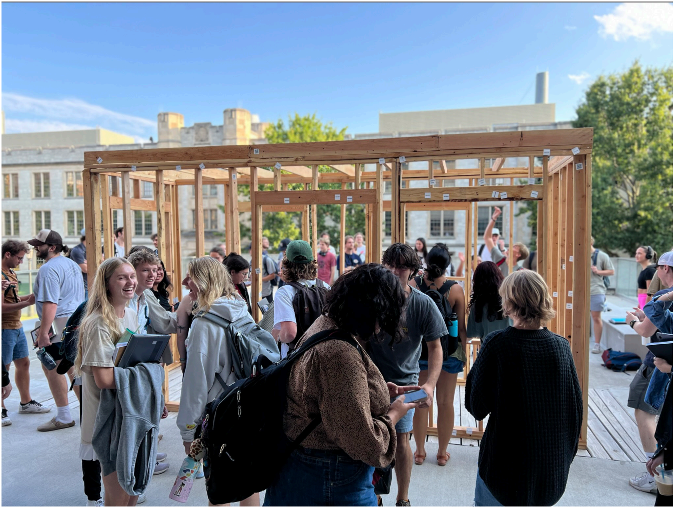
Figure 3. Completed Normative Stick Frame
